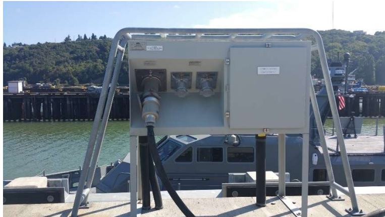
Shore Side Electricity distribution station.
