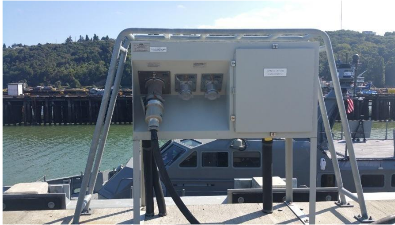
Shore Side Electricity distribution station.
